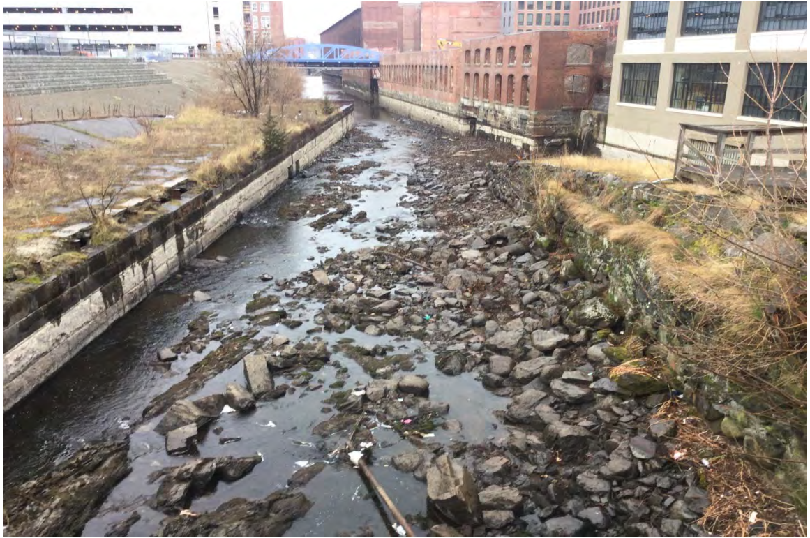
Photo 5-9. Substrate debris at the bottom of Pawtucket Canal adjacent to Appleton Mills and downstream of Swamp Locks.
