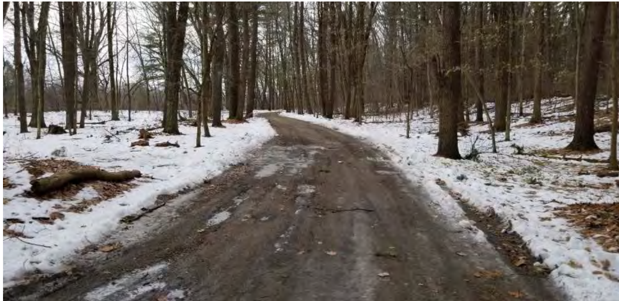
Photo 5 – Access road to Greeley Boat Ramp
