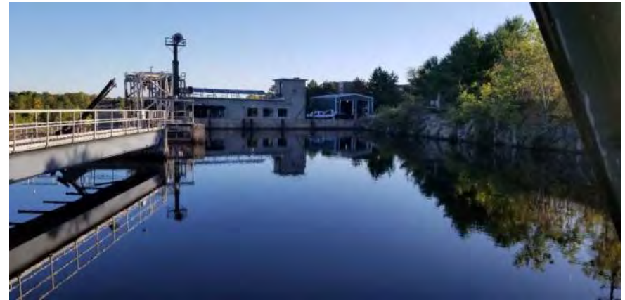
Polygon No.: 94 Photo Location No.: P-8 Date: 9/26/2019 Direction Photo Taken: Northerly Description: View looking west toward E.L. Field Powerhouse from the NPS walking trail. Vegetation is growing on bedrock along south side of the canal.
