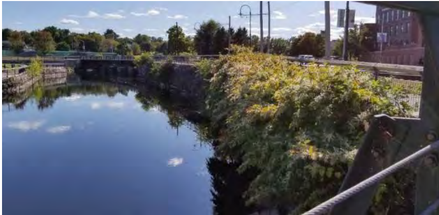
Polygon No.: 18 Photo No.: 18 Date: 9/25/2019 Direction Photo Taken: Southwesterly Description: Approximately 20 percent of the canal wall has woody trees, shrubs, and/or herbaceous plants growing on it. The vegetation includes tree of heaven, maple, common mullein, Japanese knot weed, and ragweed. Japanese knot weed coverage increases with closer proximity to the National Park Service boat dock.
