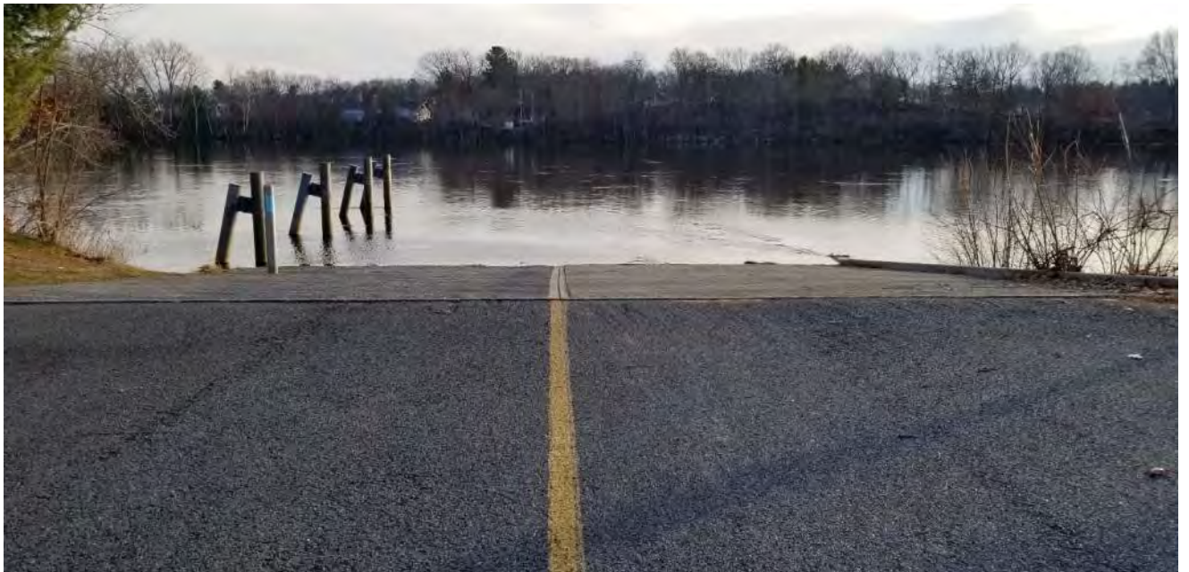
Photo 22 – Paved Rourke Brothers Boat Ramp
