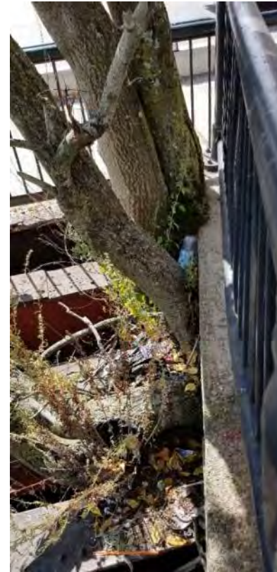
Polygon No.: 4 Photo No.: 4 Date: 9/25/2019 Direction Photo Taken: Southerly Description: There is one, multi-trunked tree of heaven tree at approximately 4 to 6 inches diameter at breast height growing out of the canal wall.
